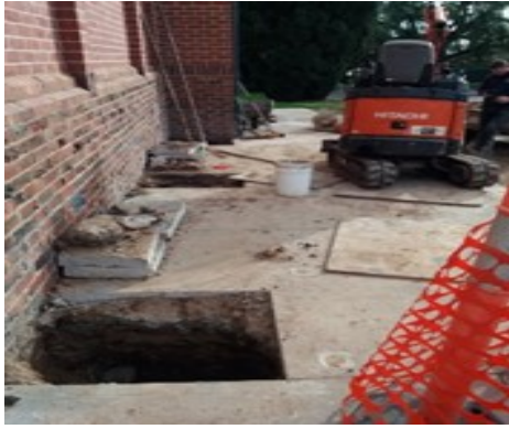
Underpinning Preparation
